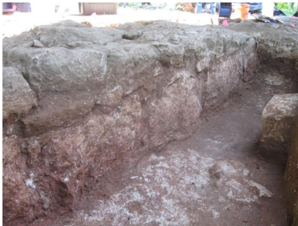
Massive stones along the East Wall
